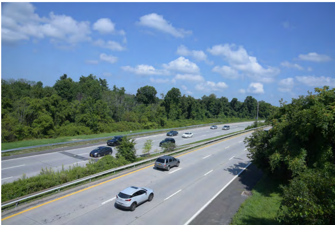
Photo 4 Sprain Brook Parkway looking northeast at the Project Site.
