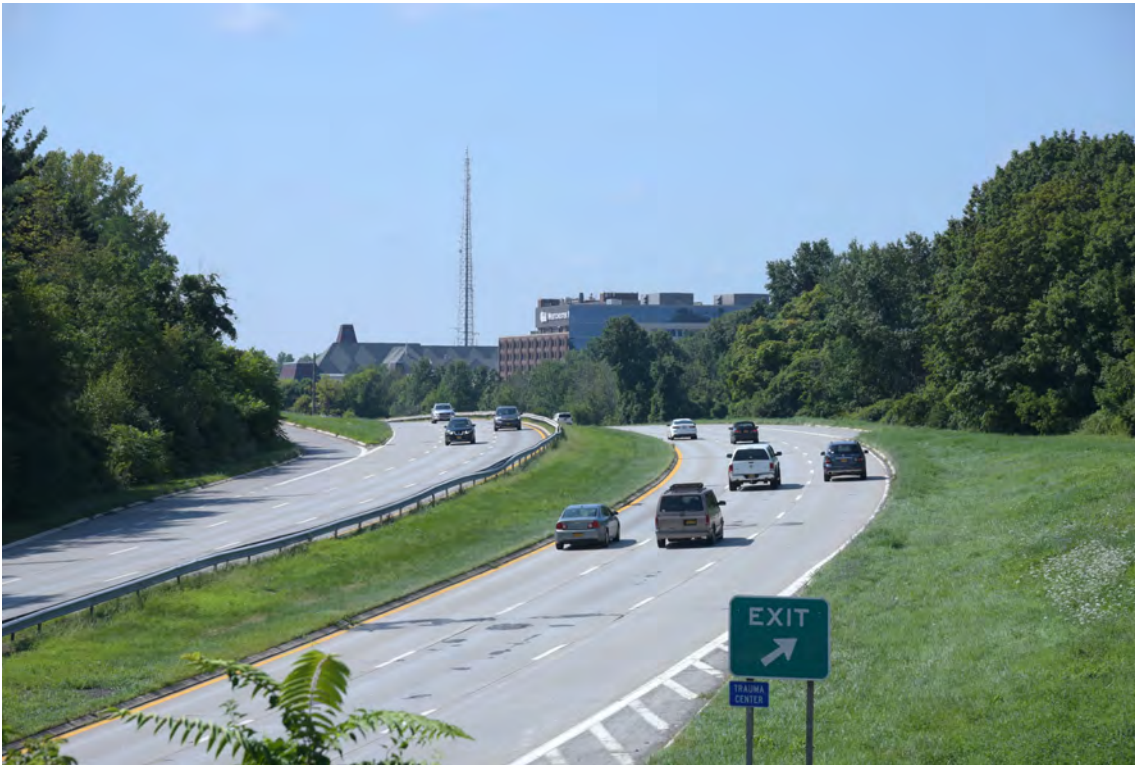
Photo 3 Looking south over the Sprain Brook Parkway at the Project Site (right) from the Bradhurst Avenue Sprain Parkway Overpass.
